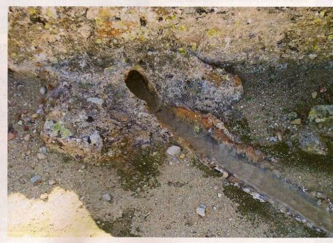
ferred the steaming-hot geothermal water to the pool complex. At the pool, these four-inch pipes had been set within coves around the perimeter of the pool, with plaster built up over them to diffuse the heat more evenly through the water. All was then topped with beautiful mosaics.
