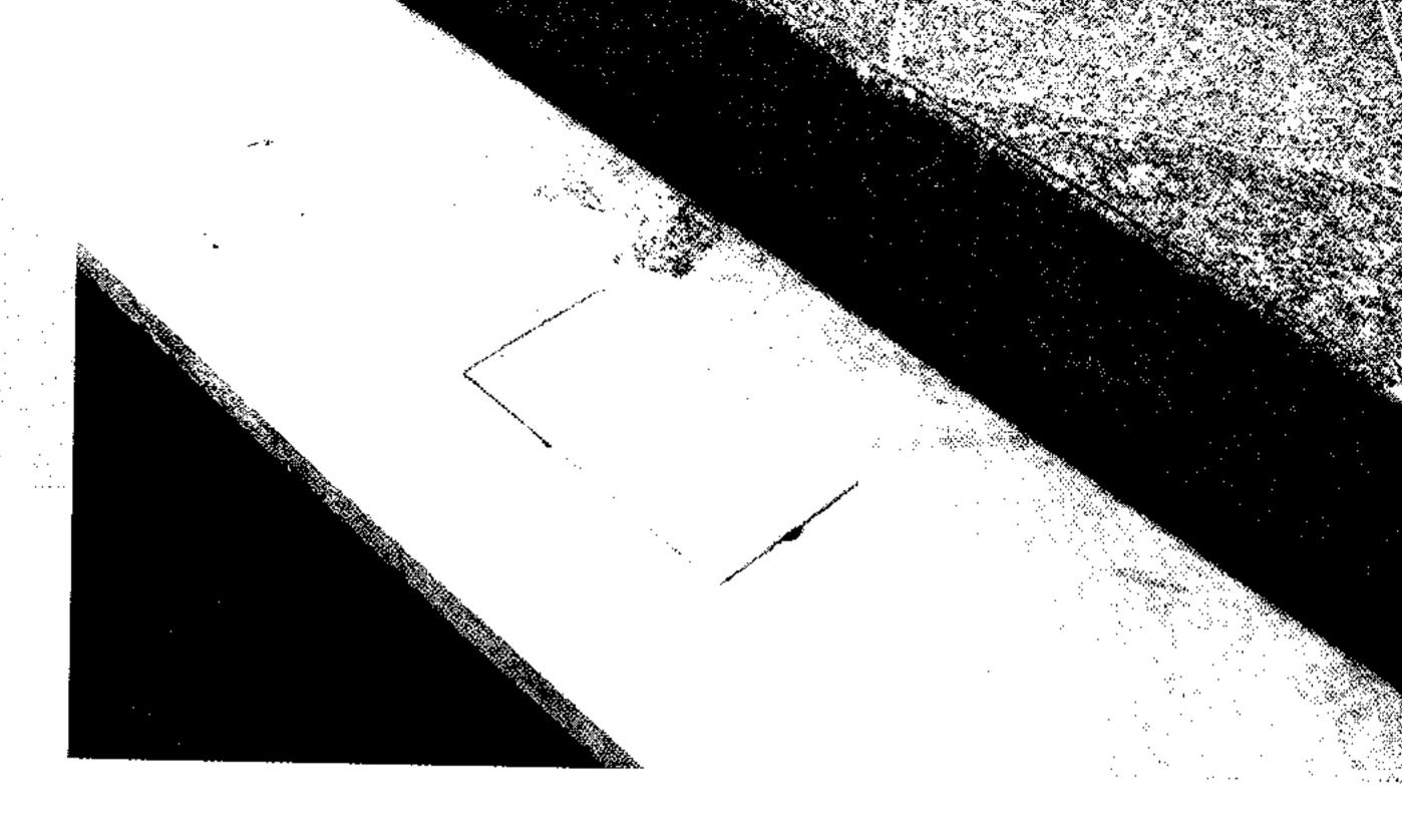
In construction, we create a small box in which we've placed two lines — one for the controller's cables and the other a drain. When the coping is installed, my masons cut out a piece of the stone over the box. This piece will eventually become a lid we make fully functional by carving out a finger cup.
